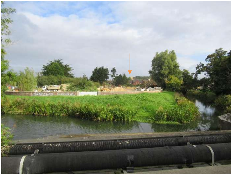
Plate 6. View towards the Parish Church of St Mary from Skilling Hill Road bridge
