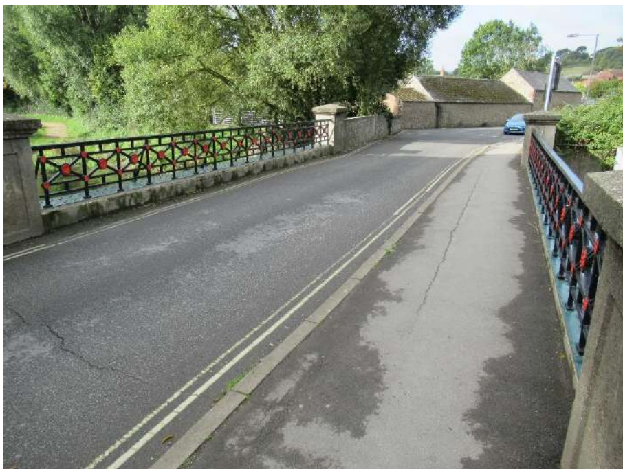
Plate 13. Skilling Hill Road Bridge
