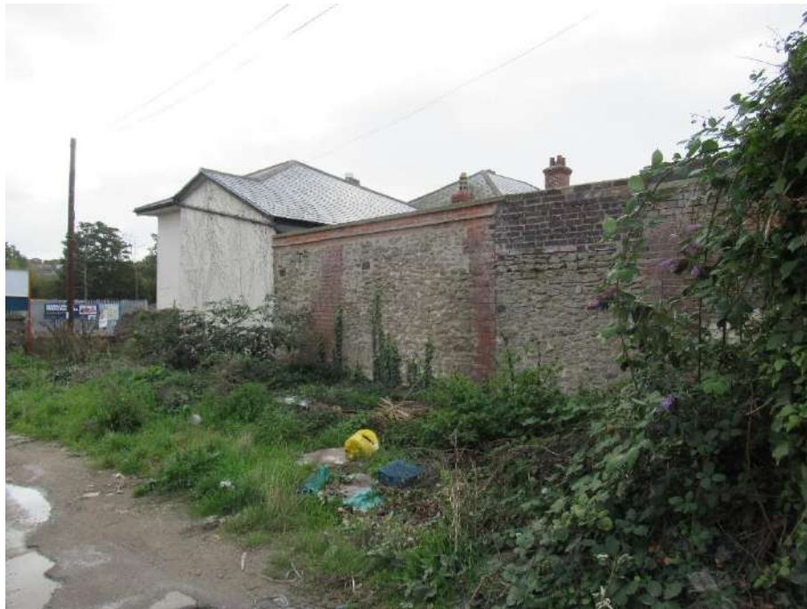
Plate 9. View towards the north elevation of 158 South Street
