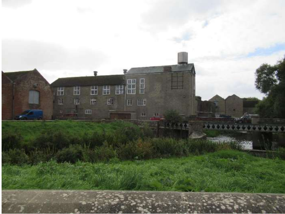
Plate 20. View towards Bridport Old Brewery from the southern extent of the Site
