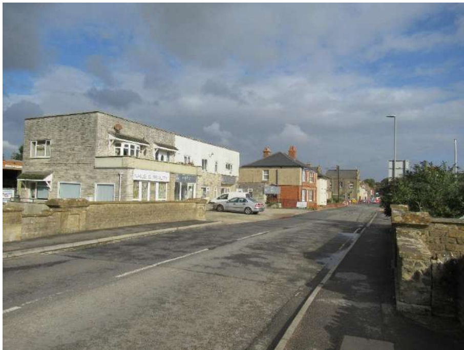
Plate 11. South Bridge looking north
